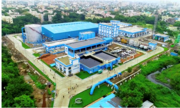
Distinction Award under "Wastewater Project of the Year" from the Global Water Intelligence for our Koyambedu TTRO Plant, Chennai
