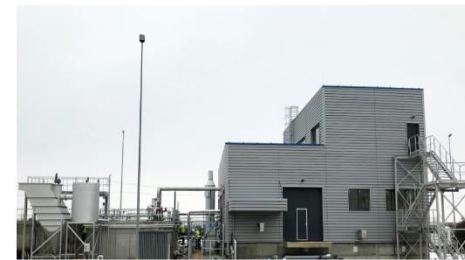
Industrial Effluent Treatment Plant for Phillip Morris, Otopeni, Bucharest, Romania Treatment of effluents from tobacco production
