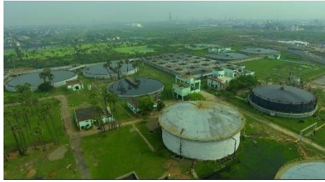
110 MLD Sewage Treatment Plant, Kodungaiyur, Chennai, India One of the most energy efficient and energy neutral STPs in the country
