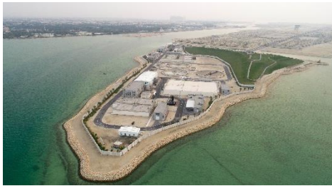
Al Madina Al Shamaliya 40 MLD Sewage Treatment Plant, Bahrain Awarded Wastewater Project of the Year at Global Water Awards, 2019
