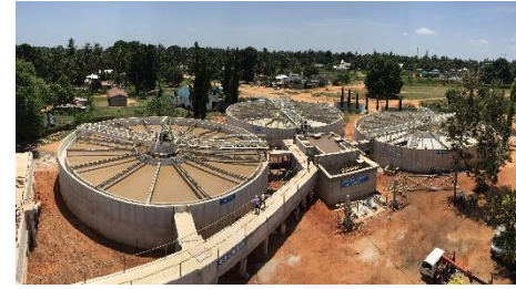
130 MLD Drinking Water Treatment Plant, Tanzania First water project in Africa to be commissioned under EXIM India funding
