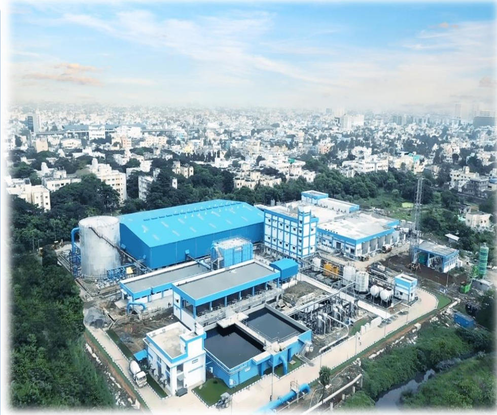
Tertiary Treatment Reverse Osmosis ('TTRO') Plant Koyambedu, Chennai, India
