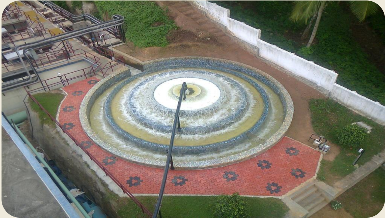
Water Treatment Plant, Meenad, Kerala
