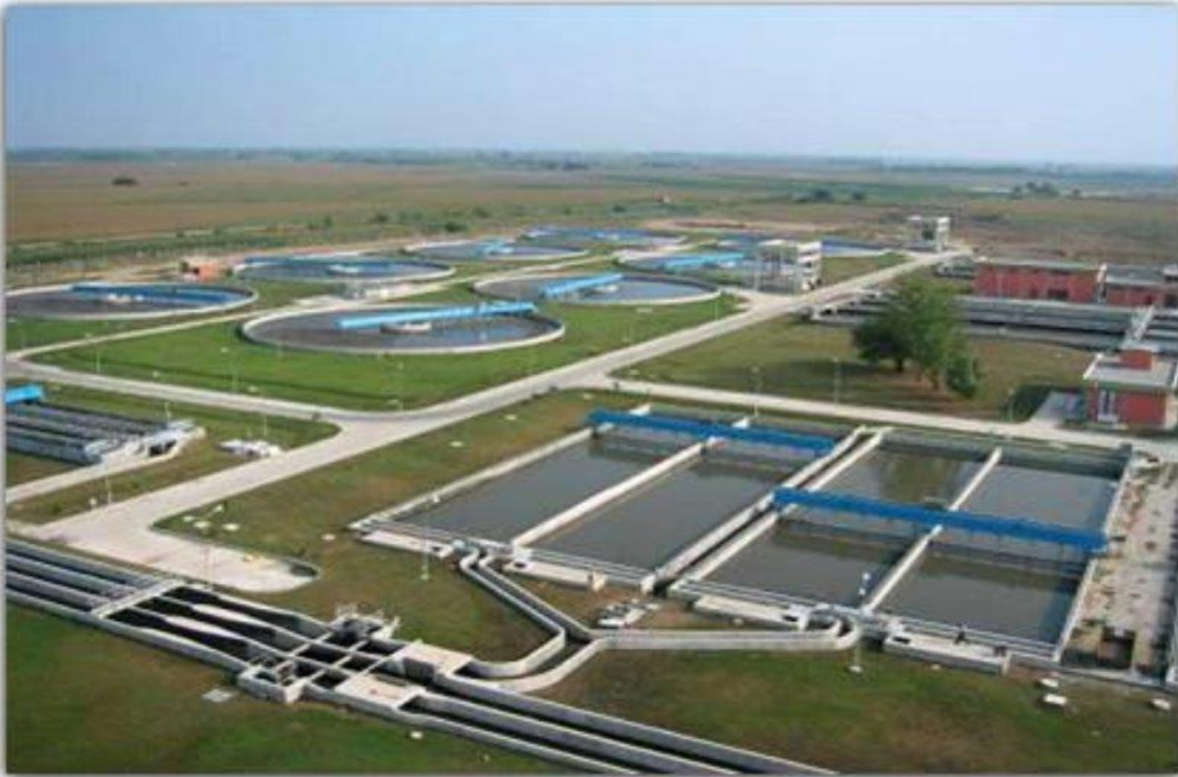
Waste Water Treatment Plant, Turkey
