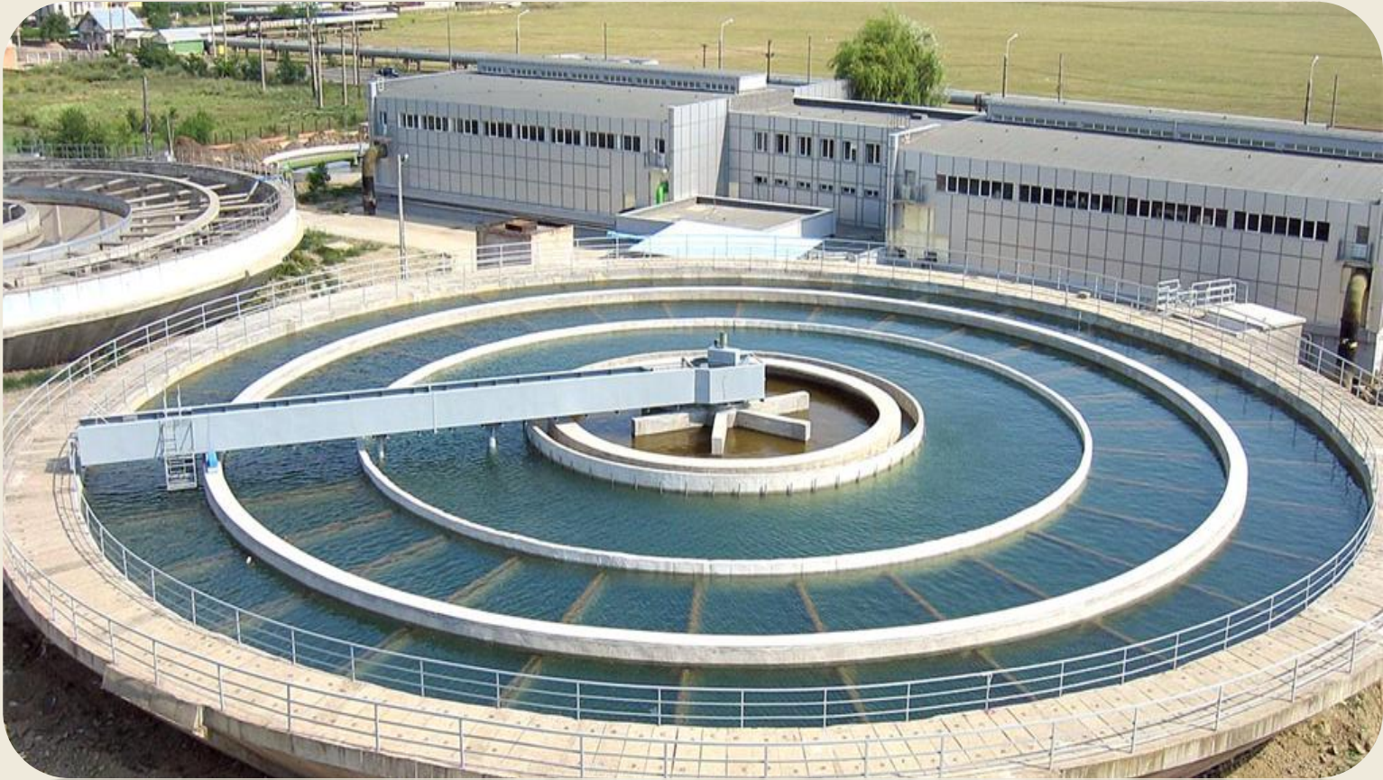
Chirita, Water Treatment Plant, Romania
