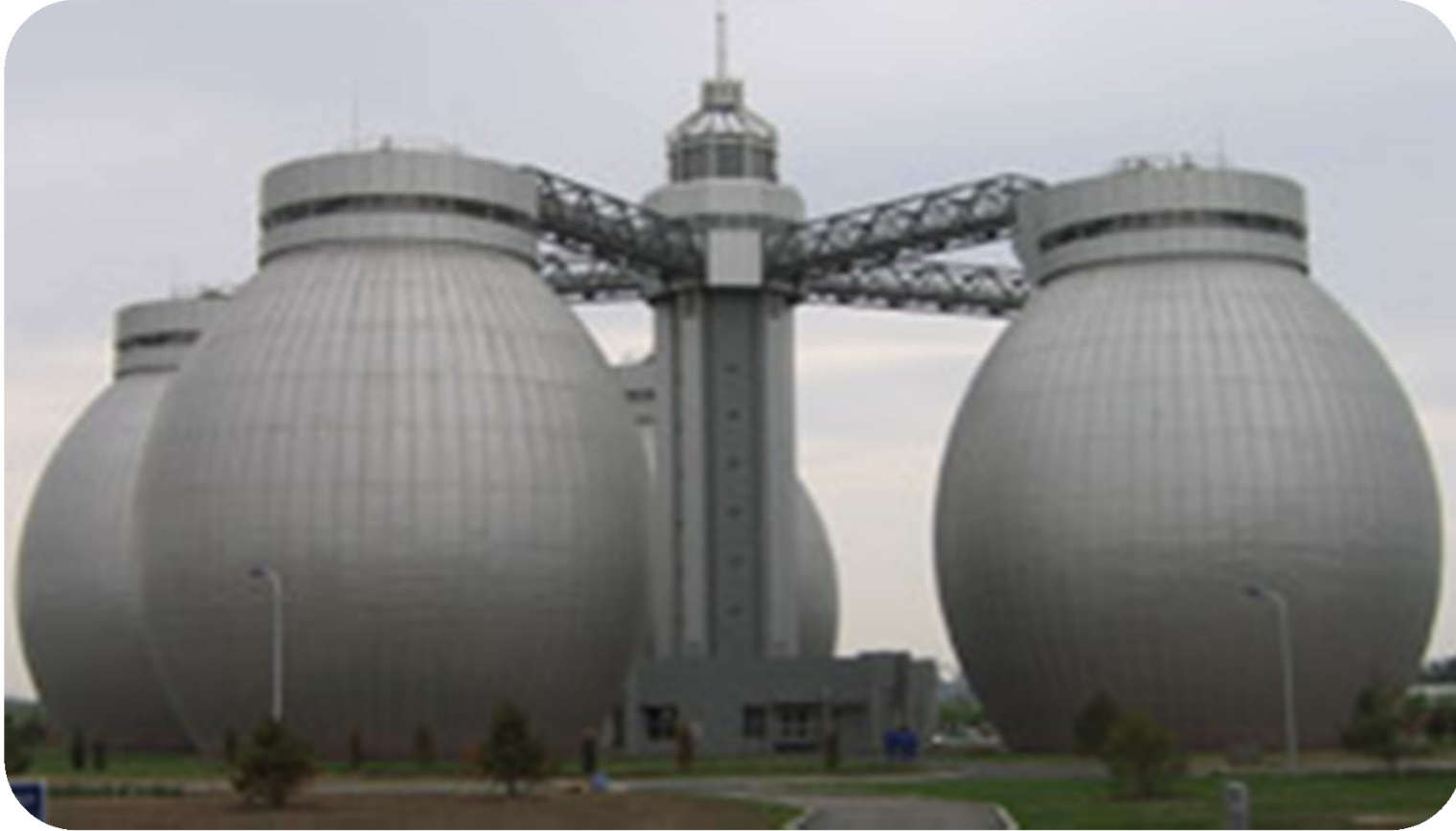
Xiaohongmen WWTP, Sludge Treatment, Beijing, China
