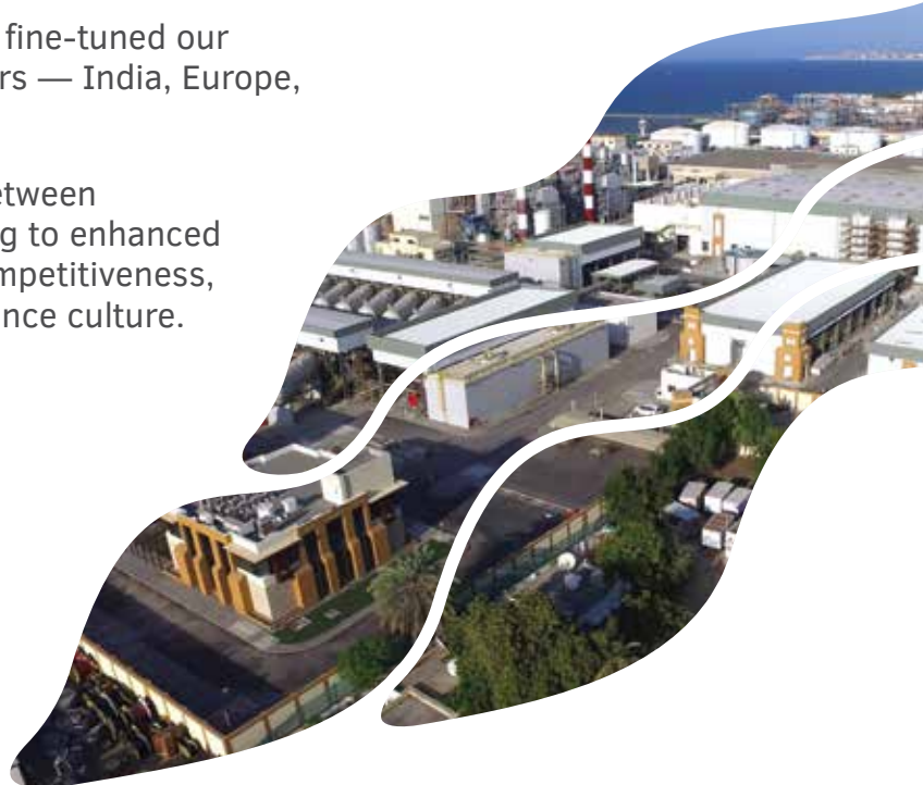
Al Ghubrah seawater desalination plant, Oman
